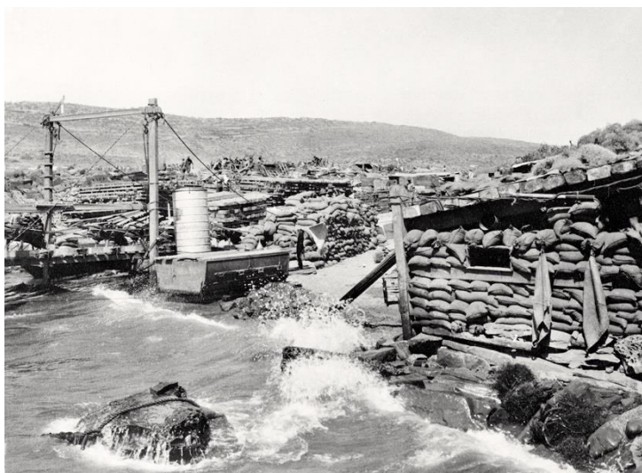
Picture: 1915 Kangaroo Beach, Suvla Bay. The 1st RAN Bridging Train served in the Gallipoli Campaign. This photo shows part of the Pontoon Pier and sandbag structures erected by the RANBT at Kangaroo Beach, Suvla Bay. Photo Credit: RAN.
