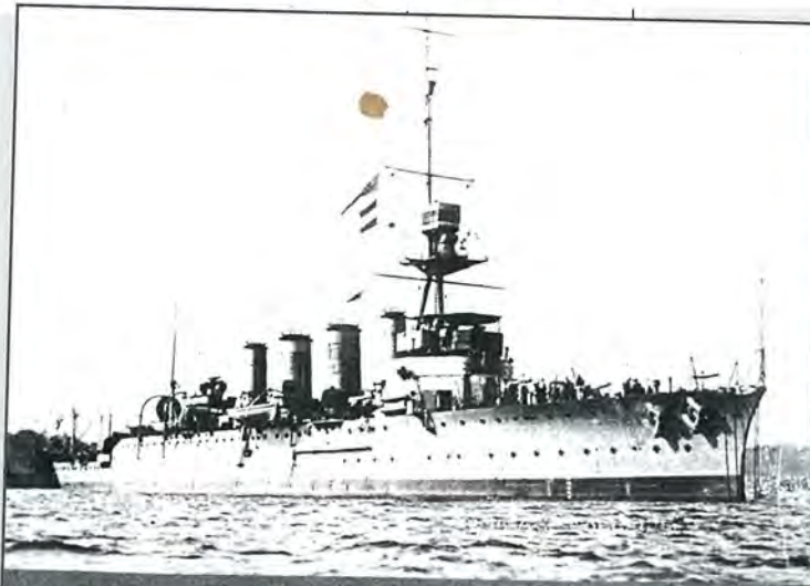
H.M.A.S. "ADELAIDE," Light Cruiser. Displacement, 5,500 tons. Horse Power, 25,000. Armament, Nine 6", One 3" A.A., One 12 Pounder and Four 3 Pounder Guns. Built by the Australian Commonwealth Naval Yard, Sydney. Completed in August, 1922.
