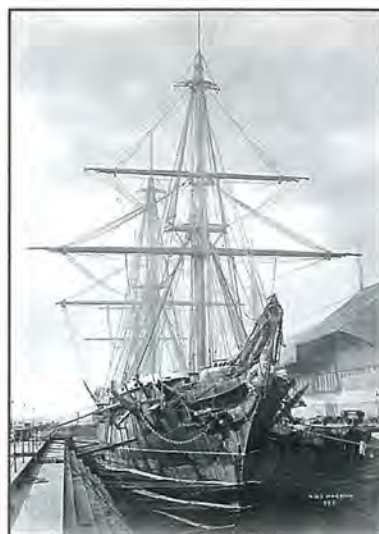
HMS Warrior marked a turning point with her iron hull and armour. Powered by both steam and sail, she featured a citadel - an armoured turret housing guns
