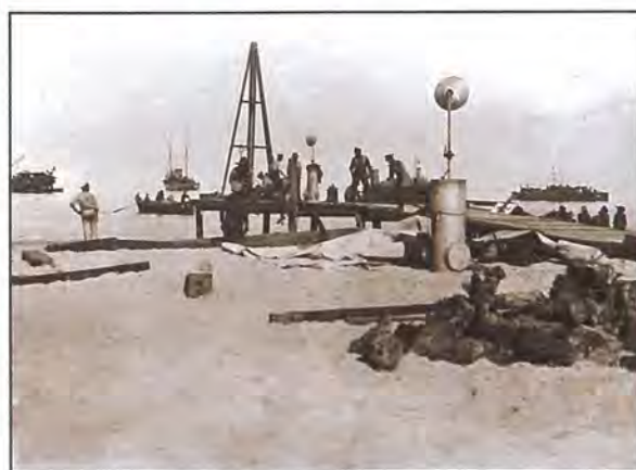
Bridging Train at El Arish in 1916 building a wharf to support the advancing ANZAC Mounted Division in its push into Palestine. The unit landed on a mined beach to build wharves to provide logistics support to advancing forces. The RANBT came under Turkish shell fire and air attack.
