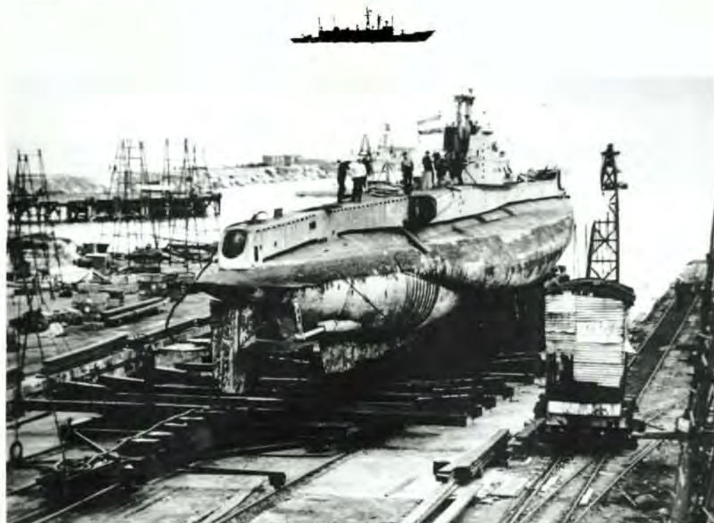
The Royal Netherlands Navy T-class submarine TIJGERHAAI (ex-HMS TARN) under refit on the Public Works Slipway in the Port of Fremantle in Western Australia in July 1946. (Photo by courtesy of Vic Jeffery)
