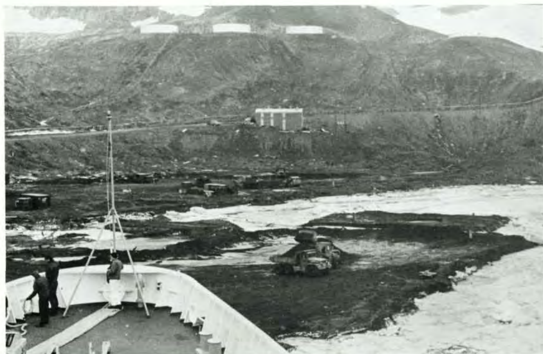
The ice wharf at McMurdo Base is covered with earth in summer to slow the melting process but too much earth will cause the wharf to sink.
